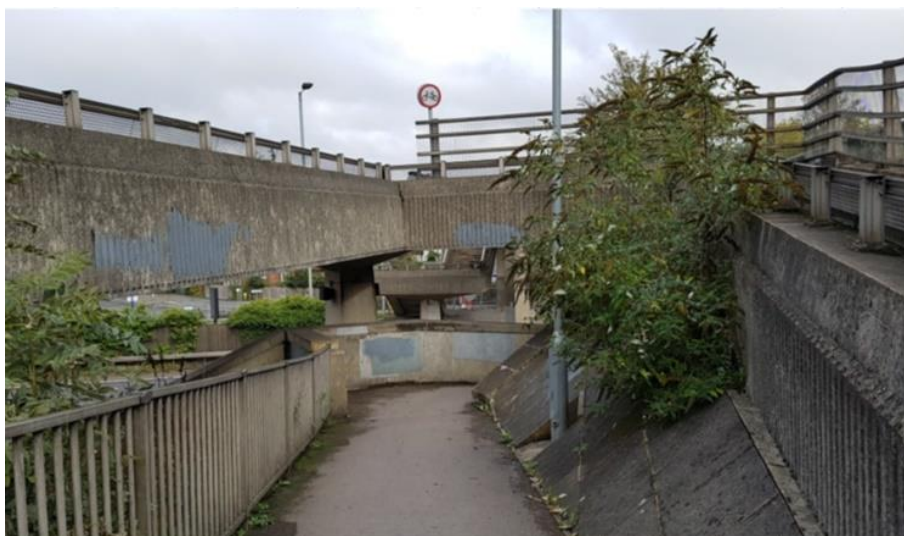
Wooden Bridge – cycling is not permitted, due to a combination of narrow deck, low balustrade/parapet and tortuous ramps/steps. All of these will need to be addressed to allow cycling as well as use by disabled people.
