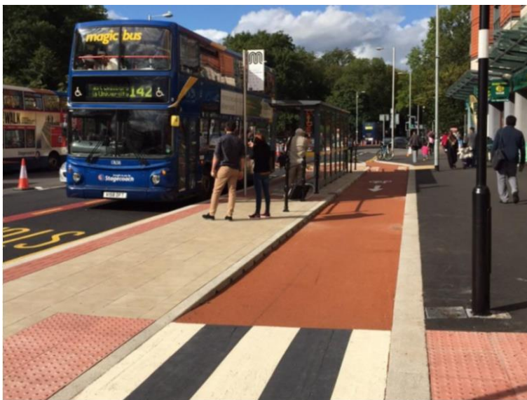
Example of a one-way segregated cycle track and floating bus stop in Manchester.
