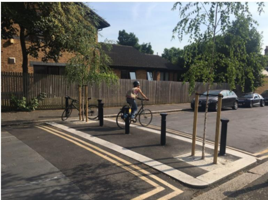
A basic modal filter with bollards and tree planting allows cyclists and pedestrians to pass through while preventing vehicle through movement
