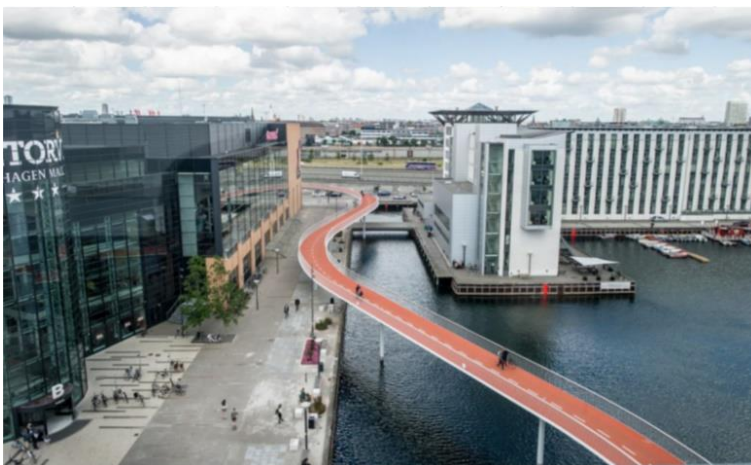
This bridge in Copenhagen known as the 'bicycle snake' provides a longer link across water bodies and through an urban area.
