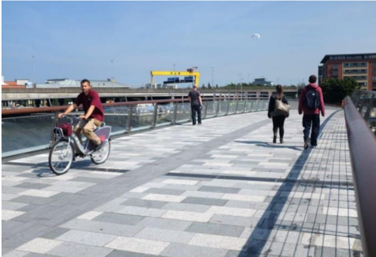
This shared pedestrian and cycle bridge provides a generously wide space and gentle gradient.
