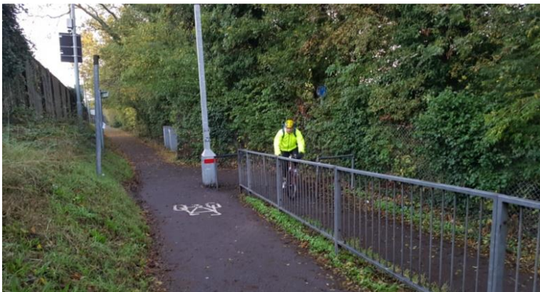
The railway bridge/A3 underpass between Southway and Perimeter Road features narrow width, difficult bends and obstructive street furniture making cycling and pedestrian conditions challenging and unattractive.
