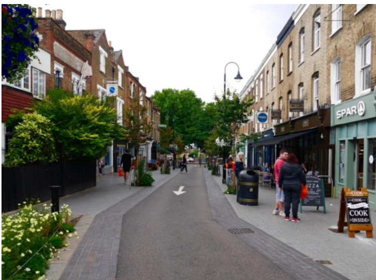
Orford Road in LB Waltham Forest uses a camera enforced bus gate to restrict through-traffic and enable public realm improvements on a local neighbourhood high street.
