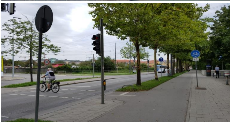
Example of a two-way or bi-directional cycle track in Munich and pedestrian and cycle crossing facility. Here, a planted strip acts as a buffer between the carriageway and cycle track. A change in materials indicates separation between the footway and cycle track.
