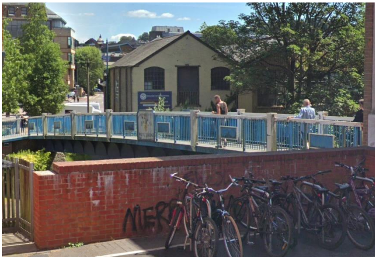
Walnut Bridge crosses the River Wey Navigation, linking Walnut Tree Close and the Bedford Wharf area. It is currently narrow with steep ramps. Guildford BC has agreed proposals to replace the bridge. The new bridge will have a wider deck and allow use by both pedestrians and cyclists. It will also have a more accessible ramp allowing easier use by disabled people.
