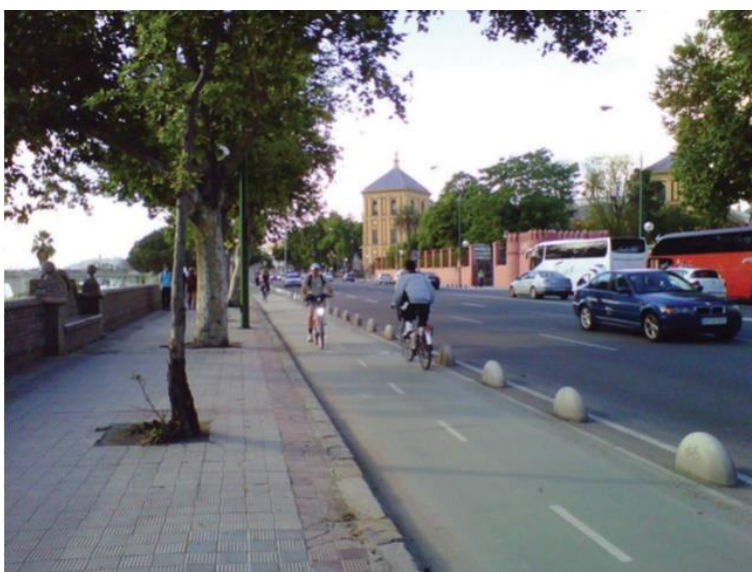
Example of a two-way or bi-directional cycle track in Seville using light segregation.
