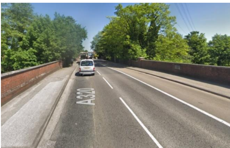
Woking Road features this bridge across the River Wey and River Wey Navigation. Introducing cycle facilities here while retaining the footways and bus lane would require widening the bridge by approximately 3-4m. The bridge is used heavily by school children walking and cycling and would form part of the route between the town centre and Slyfield Industrial Estate and the new Slyfield Area Regeneration Area.
