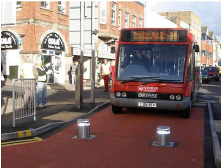
A bus gate using automatic rising and falling bollards.
