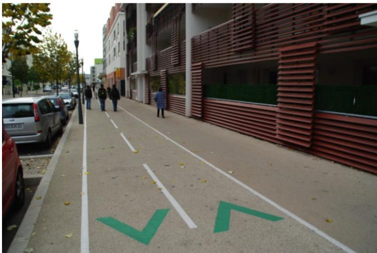
Example of a 2-way footway level cycle track in Marseille, illustrating different levels of segregation between cyclists and vehicles and cyclists and pedestrians.
