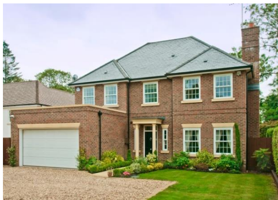
5 bed 'Re-build' following demolition of small bungalow, 2012
