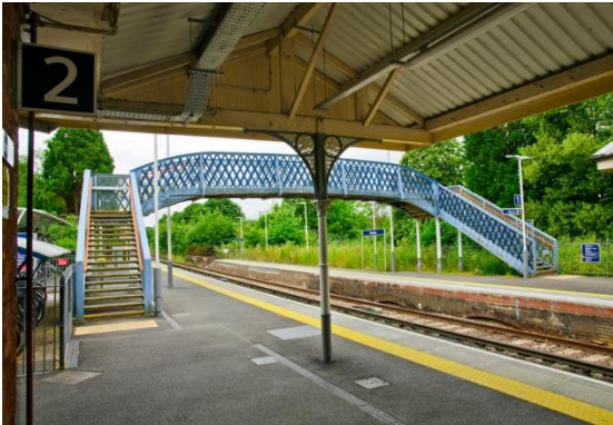
Footbridge at Horsley Station: not wheelchair accessible
