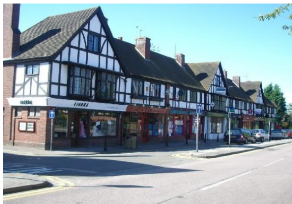
One section of Station Parade shopping area
