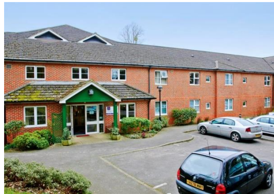
Limegrove Care Home, 55 rooms, managed by Anchor
