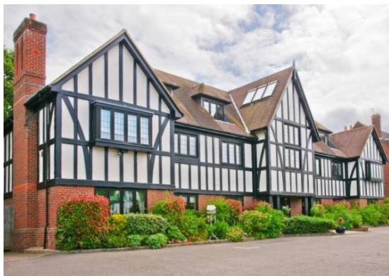
Modern style apartments, Station Parade, (2000's)
