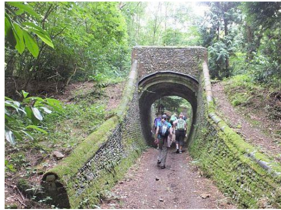
Retaining walls at Raven Arch on the Lovelace Bridges Trail
