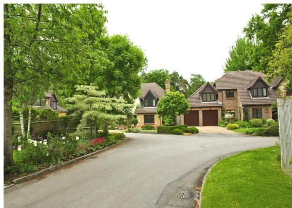
Falconwood, a backland development in the grounds of a number of large houses on Forest Road, 14 homes built in several phases.
